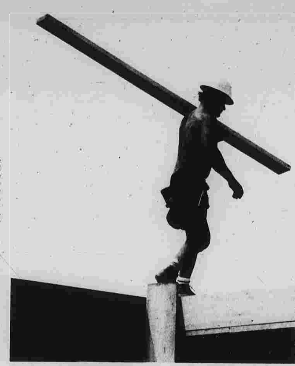
Stripped Down For Work
